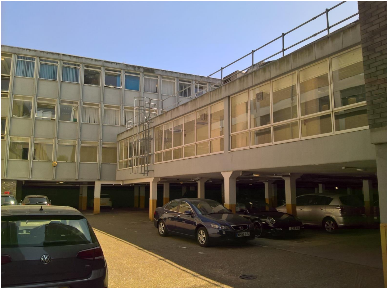
Rear of existing front tower and raised ground floor
